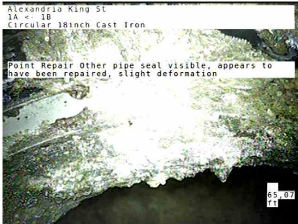
5, 00:04:24, 65.07ft Point Repair Other / pipe seal visible, appears to have been repaired, slight deformation
