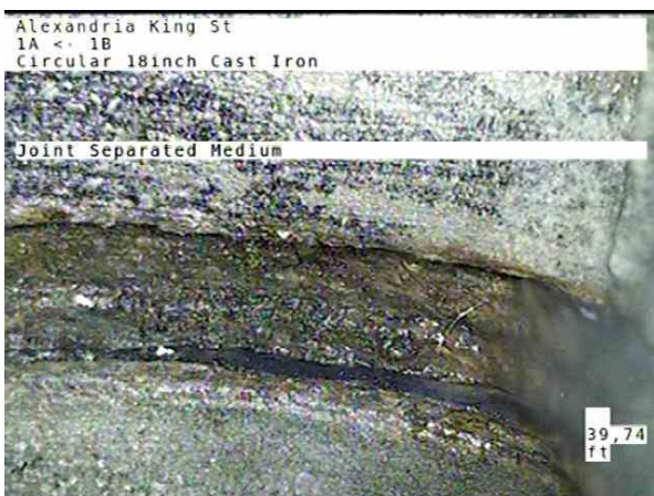
3, 00:02:34, 39.74ft Joint Separated Medium
